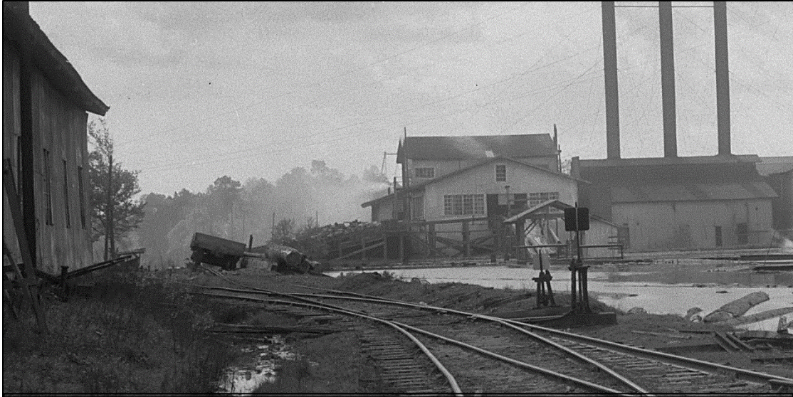
In an enlargement of the previous view, you can see the gondola perched on the end of the leaning log unloading track and the switches leading to the unloading track, as well as the connecting track leading down the hill to the Missouri Pacific line.
