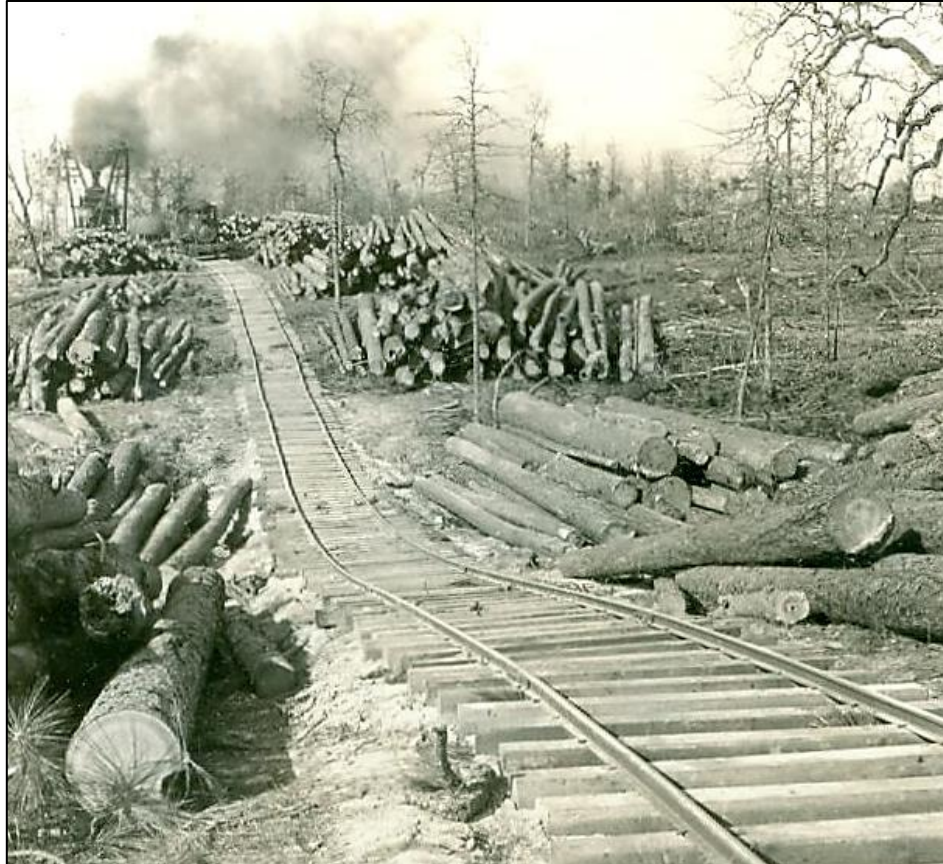
Logs skidded to the rail track by a Clyde skidder are ready for loading on log cars with a McGiffert loader. Photo by George Gerhart of the U.S. Forest Service in March 1939 (Everett 2021).
