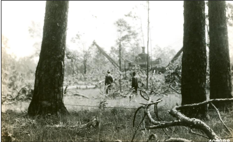
Men of the skidder crew watch a from a safe distance as it works. Note the cable between the trees in the foreground, this is a rehaul skidder. Men and animals did not have to pull the cable out to the logs—they did have to set the tongs. Working the skidder was hazardous duty. Photo by George Gerhart of the U.S. Forest Service in March 1939 (Everett 2021).
