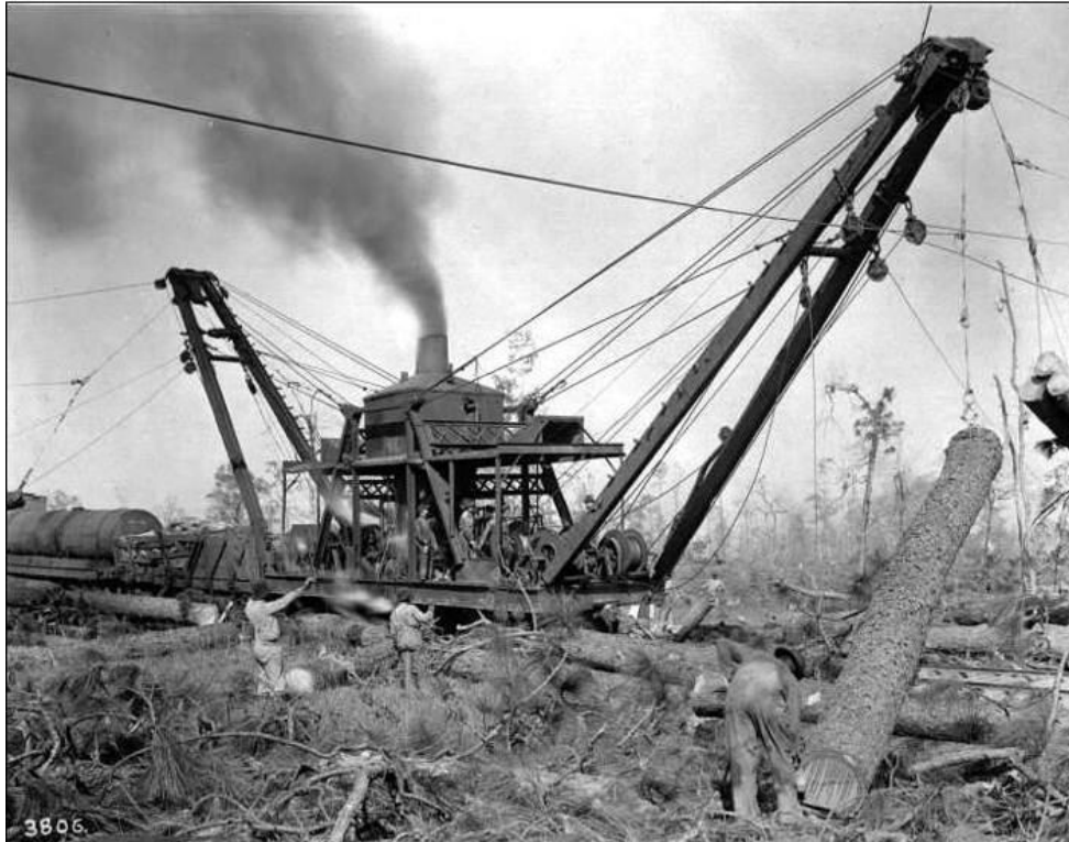
This Clyde skidder in operation shows the extent of the cabling extending out in four directions. Logs could be pulled from a 40-acre area when located at one setting on the rail track.
