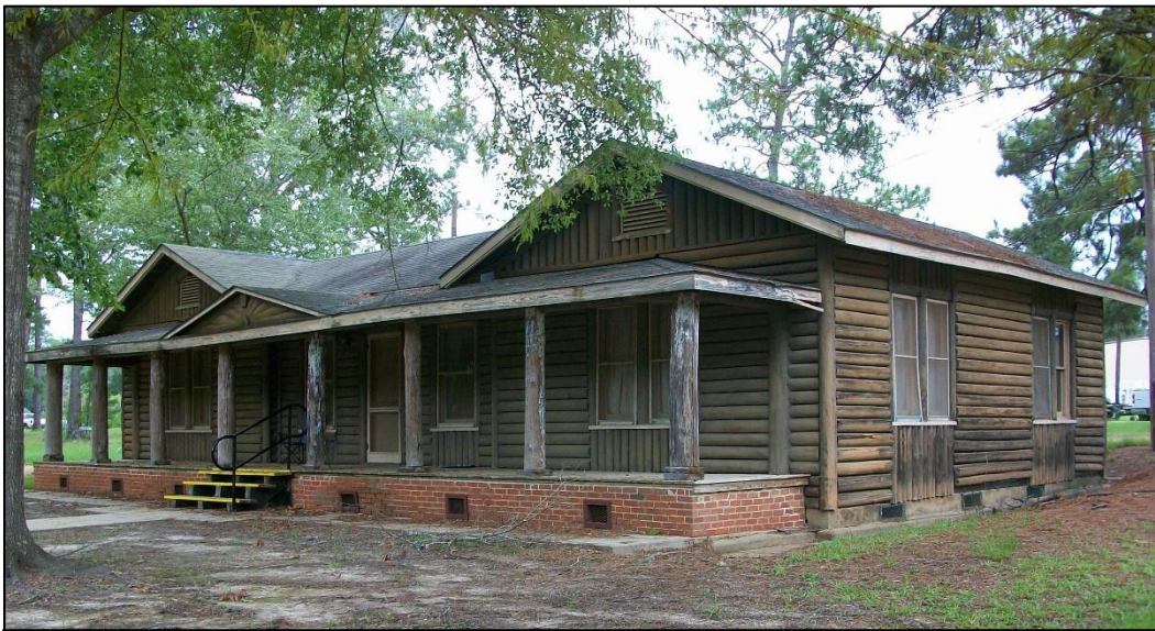
The Civilian Conservation Corps built Lech Lodge served as the headquarters for the CCC camp and later the State Forest. This photo was taken before the building was donated and moved to the Southern Forest Heritage Museum about 2012.
