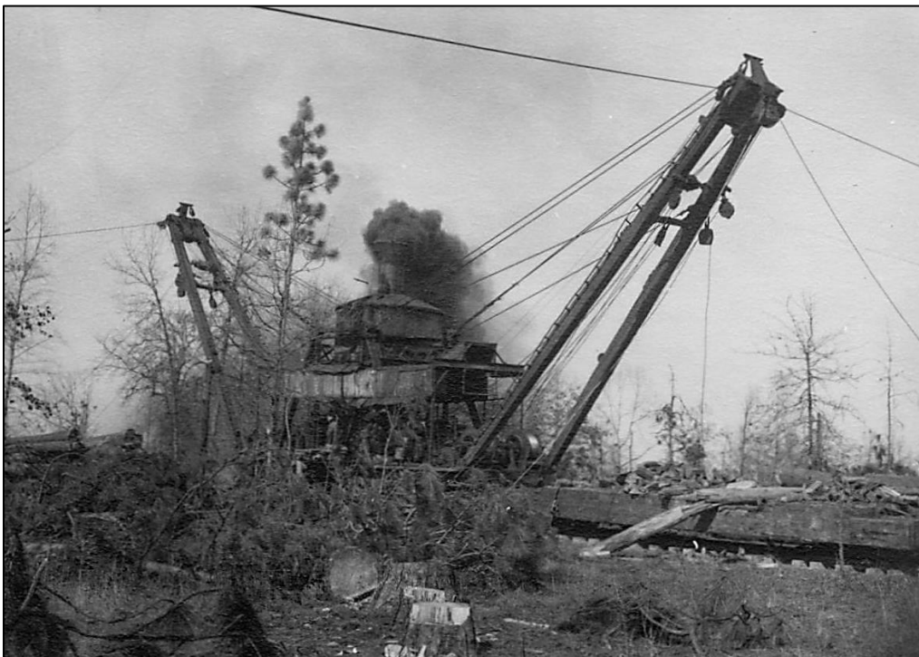
A close up of the skidder at work and the cabling involved. Notice the idler car stacked with chains, blocks, and tools. Meridian had three skidders at the time.
